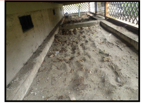
Foundation wall with exposed footing. (left side of photo)
